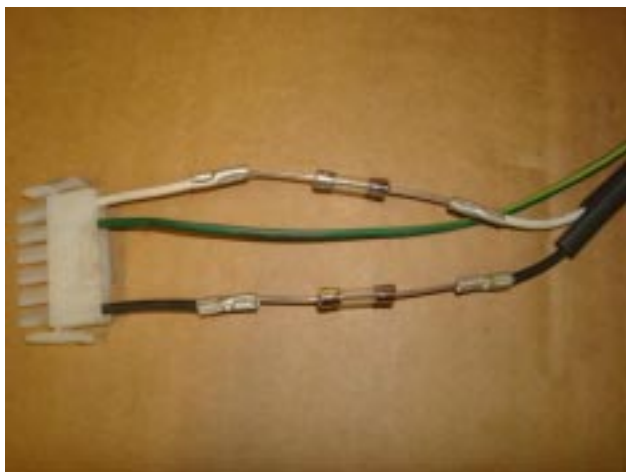
Photo 5 Install fuses with crimp connectors
