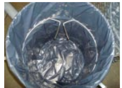
Photo 11 Install bag retainer ring
