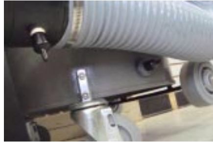
Photo 7 Fittings capped off
