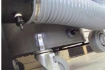
Photo 7 Fittings capped off
